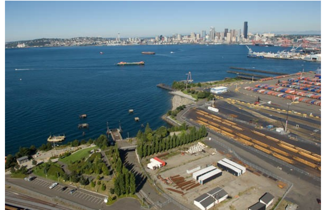
Pier 2 and Jack Block Park
